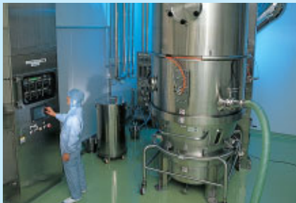
Producing Granulated Form Facility
